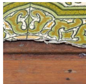
Sheet vinyl floor covering
