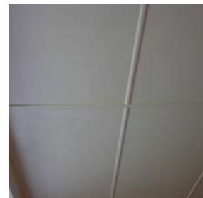
Internal wall/ceiling sheets
