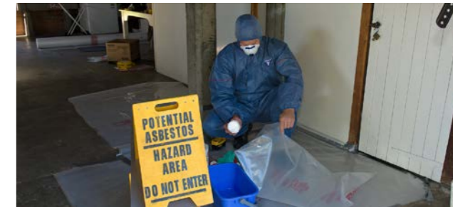
Asbestos dust control measures
