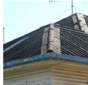
Super Six roof sheeting and guttering
